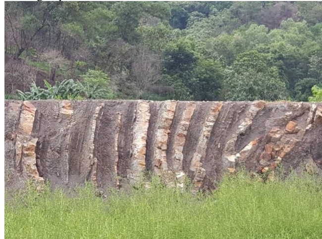
Figure 1 Exposed Rock Slope with Sub-vertical Bedding
